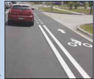
The buffer is placed between the bike lane and travel lane. The buffer is marked with two white lines to indicate the bike lane is a special use lane for bicyclists, and motorists must yield to traffic in the lane before merging or turning across the lane.
